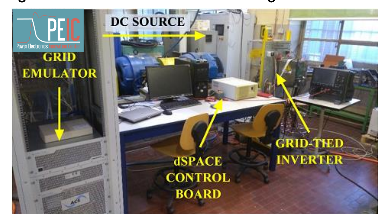
Fig 5. View of the experimental setup. The grid emulator is used to perform tests under emulated grid fault conditions.
